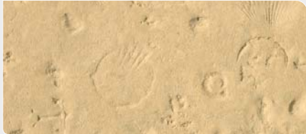
Textured Imprint Mats Large stamping mats that can be pressed into wet concrete to create unique patterns and designs.
