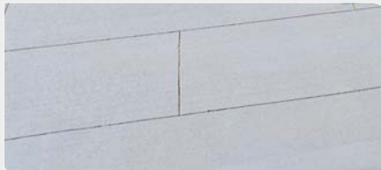
Saw Cuts or Grooved Lines Create geometric patterns with grooved joint lines in wet concrete, or by cutting the surface with a concrete saw once it has cured.
