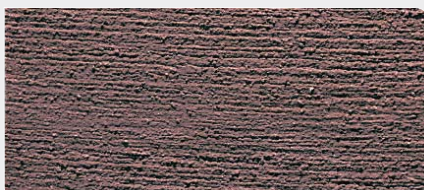
Broom Finishes Broom finishes create a textured, lineal appearance for areas requiring additional surface texture.
