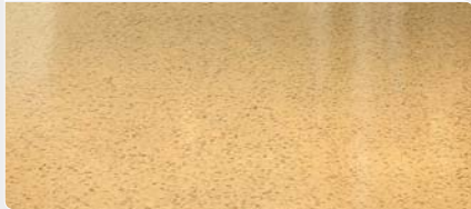
Polished Concrete The concrete surface is mechanically honed and then polished using fine abrasives. The surface result is extremely glossy and reflective.
